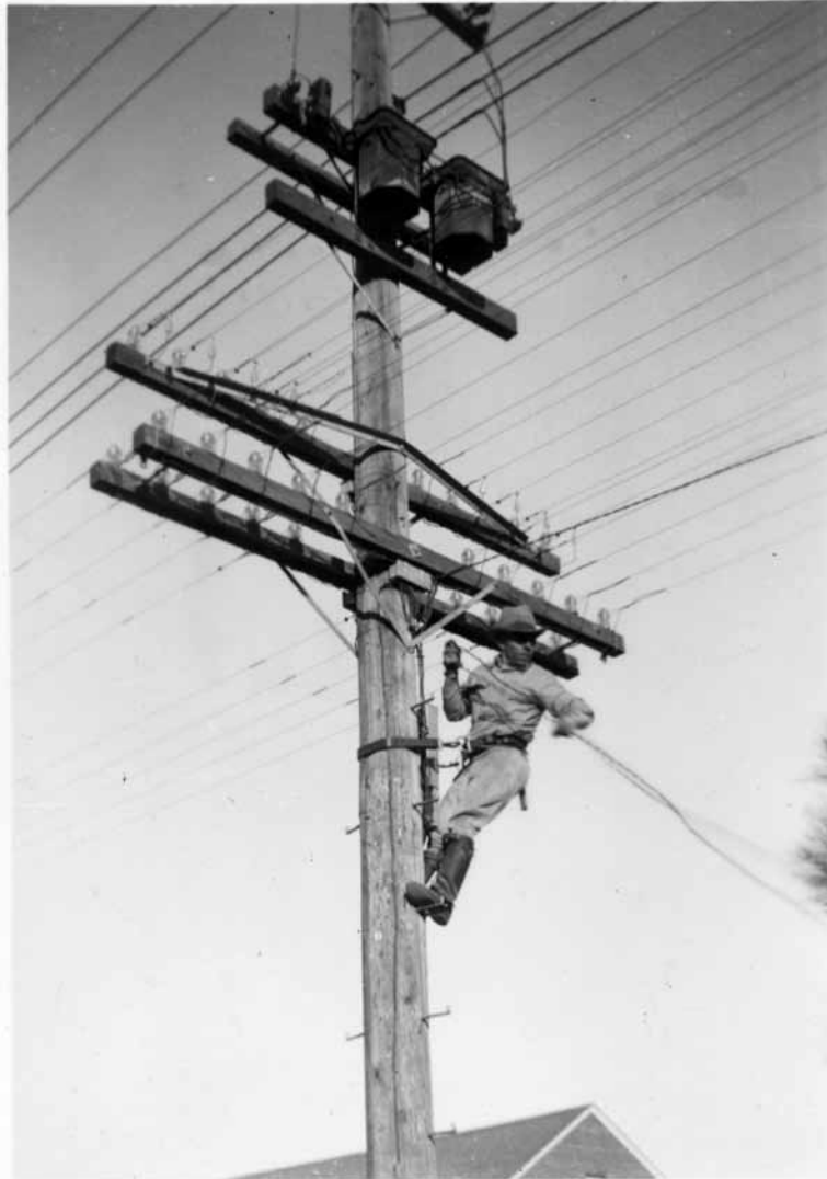
Man on telephone pole works on changing the lines, ca. 1940.
